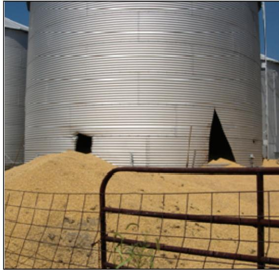
**Figure 4. One of the additional holes cut during the case study rescue (left) and the triangle-shaped opening through which the victim's body was eventually removed (right).**
