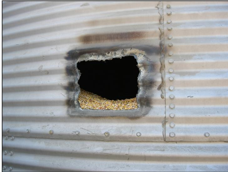
**Figure 3.** First hole cut in the bin wall during the attempted rescue documented in the case study.
